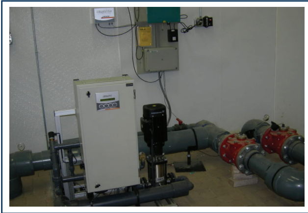
Figure 4. Fertilizer injection system
